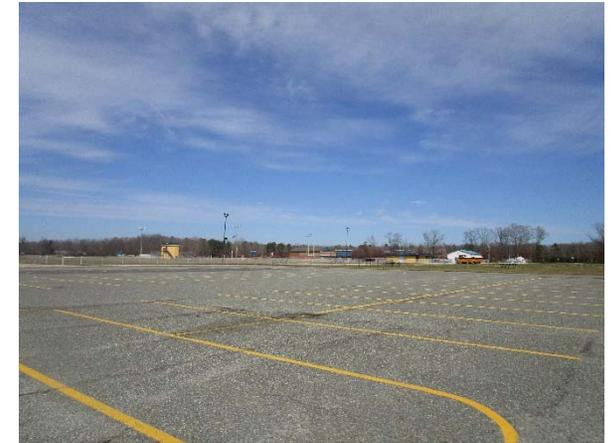
A rain garden can be installed at the corner of one section of parking lot to capture, treat, and infiltrate the associated stormwater runoff. The most southern row of parking spaces can be replaced with pervious pavement to capture and infiltrate stormwater. A preliminary soil assessment suggests that the soils have suitable drainage characteristics for green infrastructure.
