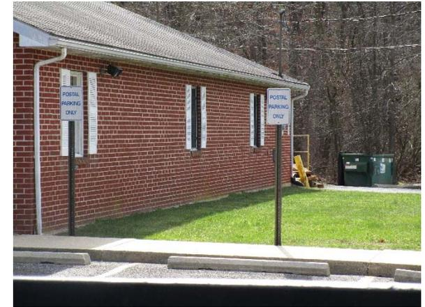
A rain garden can be installed on the northwest side of the building to capture, treat, and infiltrate rooftop runoff. The row of parking spaces closest to the building can be replaced with pervious pavement to capture and infiltrate stormwater. A preliminary soil assessment suggests that the soils have suitable drainage characteristics for green infrastructure.
