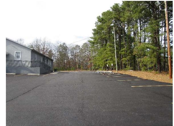
The southern half of parking spaces northeast of the building can be replaced with pervious pavement to capture and infiltrate stormwater. A preliminary soil assessment suggests that the soils have suitable drainage characteristics for green infrastructure.
